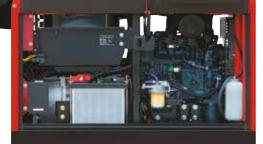
Lockable single-side service access with battery lockout. All components of the generator and diesel engine are readily accessible, and replacing filters and other consumables is simple. External drains are conveniently placed for easy access.
